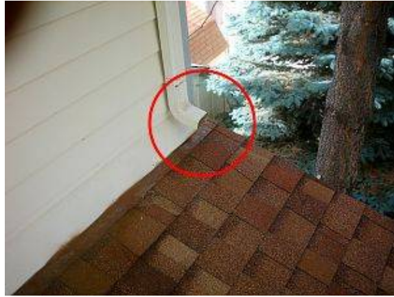
Photo 8 downspout above roof
