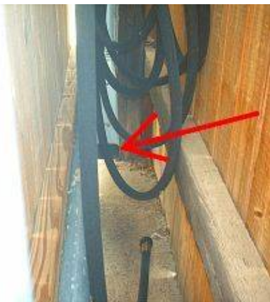
Photo 3 downspout between two fence sections
