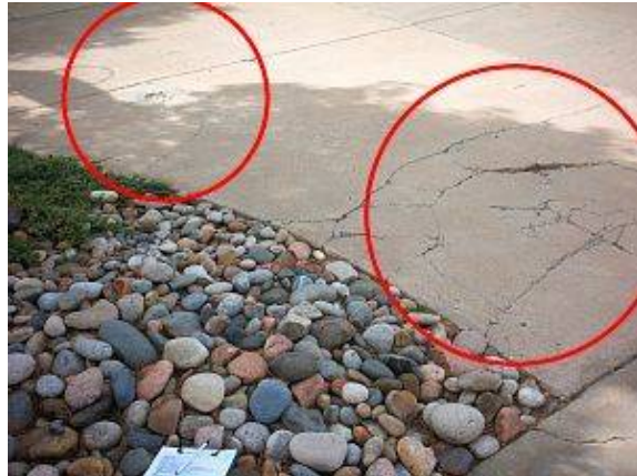
Photo 2 driveway deterioration
