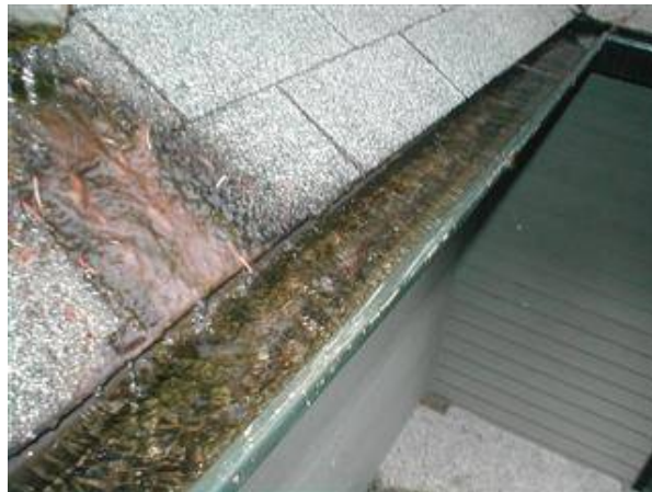
Photo 5 Overflowing gutter.
