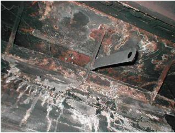
Photo 40 View up fireplace damper.
