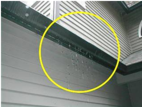
Photo 2 Overflowing gutters.
