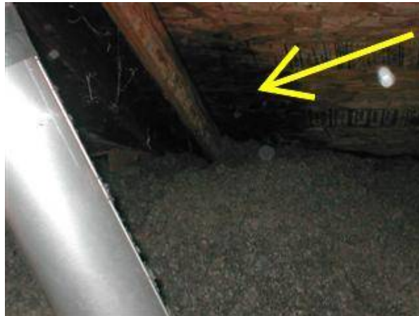
Photo 22 Blackened sheathing by wooden chimney enclosure.
