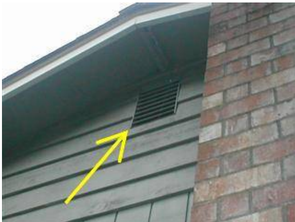
Photo 10 Gable end vent.
