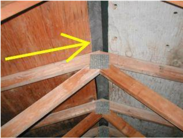
Photo 29 Slot for continuous ridge vent, viewed from attic.
