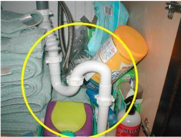
Photo 36 S-trap at upstairs bathroom sink drain.
