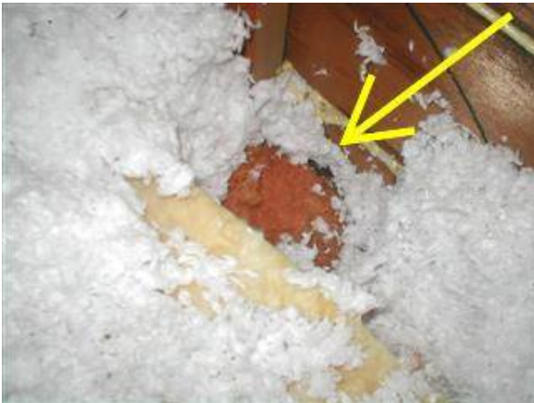
Photo 30 Silva wool insulation below newer loose fill fiberglass insulation in attic.
