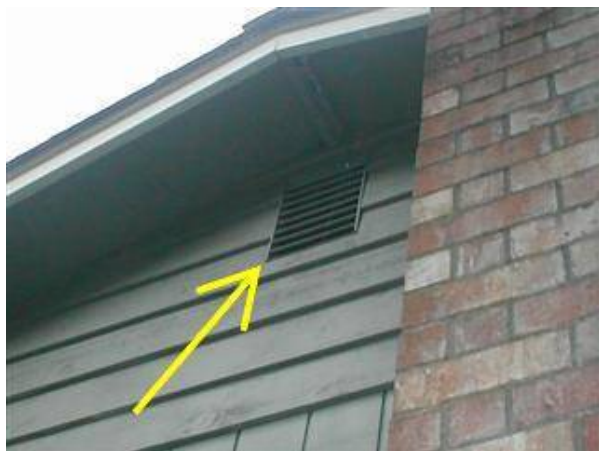
Photo 10 Gable end vent.
