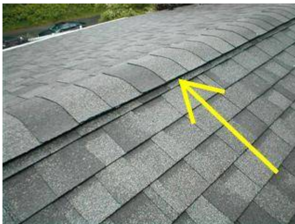
Photo 23 Continuous ridge vent.
