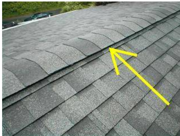
Photo 23 Continuous ridge vent.
