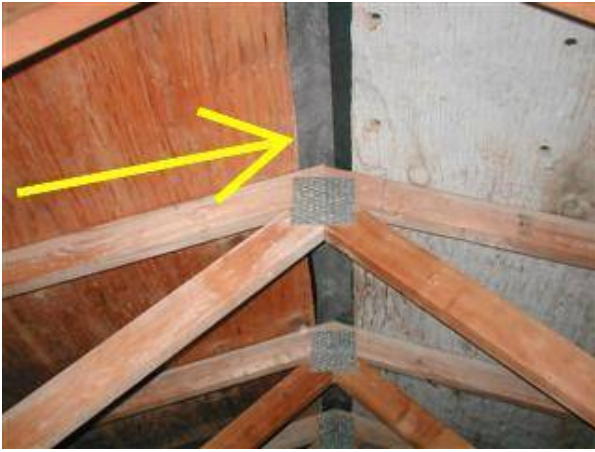
Photo 29 Slot for continuous ridge vent, viewed from attic.
